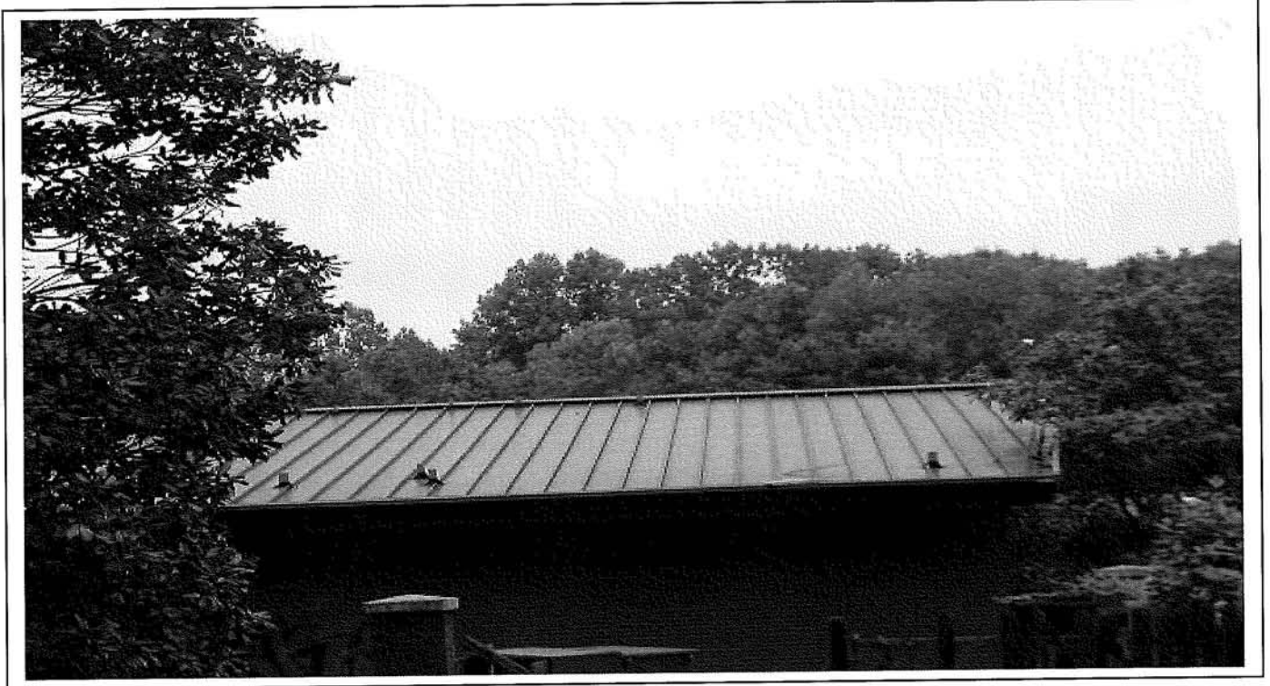
Photo 42: Typical metal raised rib roof system (all buildings)
