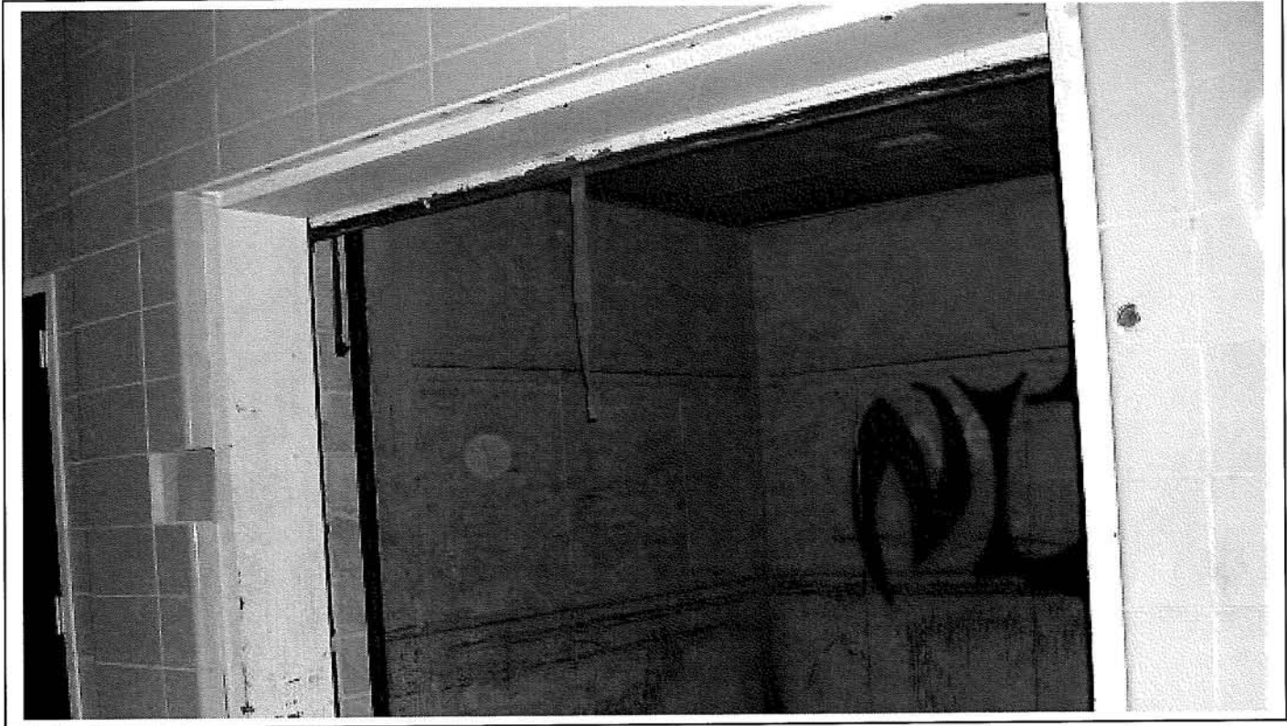
Photo 43: Typical service elevator interior (Therapy Building-Kitchen Area)
