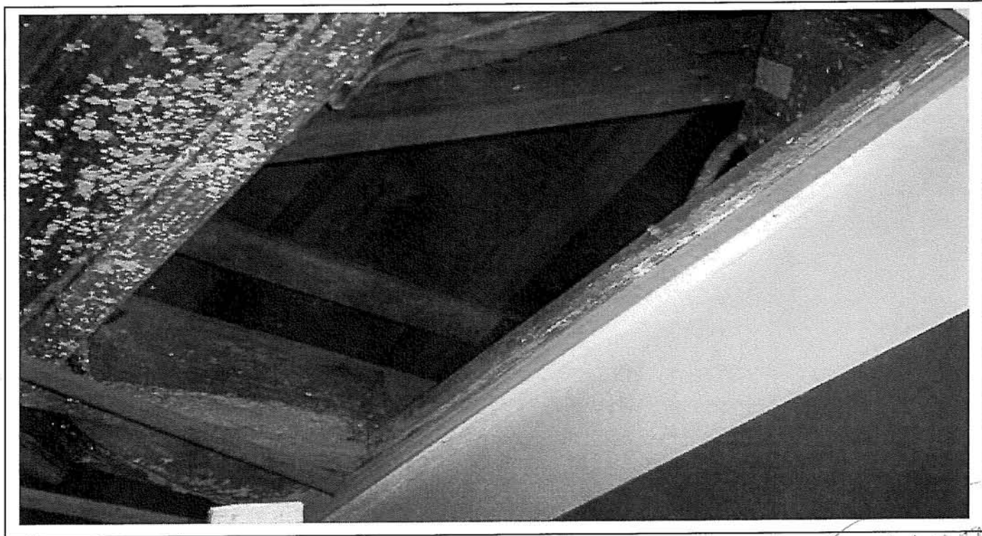
Photo 8: Structural steel I-beam with Spray-applied Fireproofing containing ACM.
