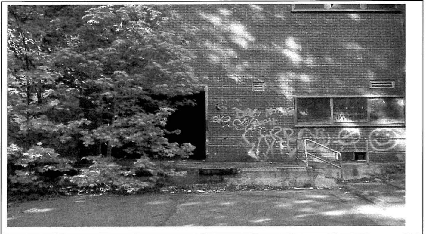
Photo 108: Exterior brick facade of ramp area, section 1 of Therapy building.
