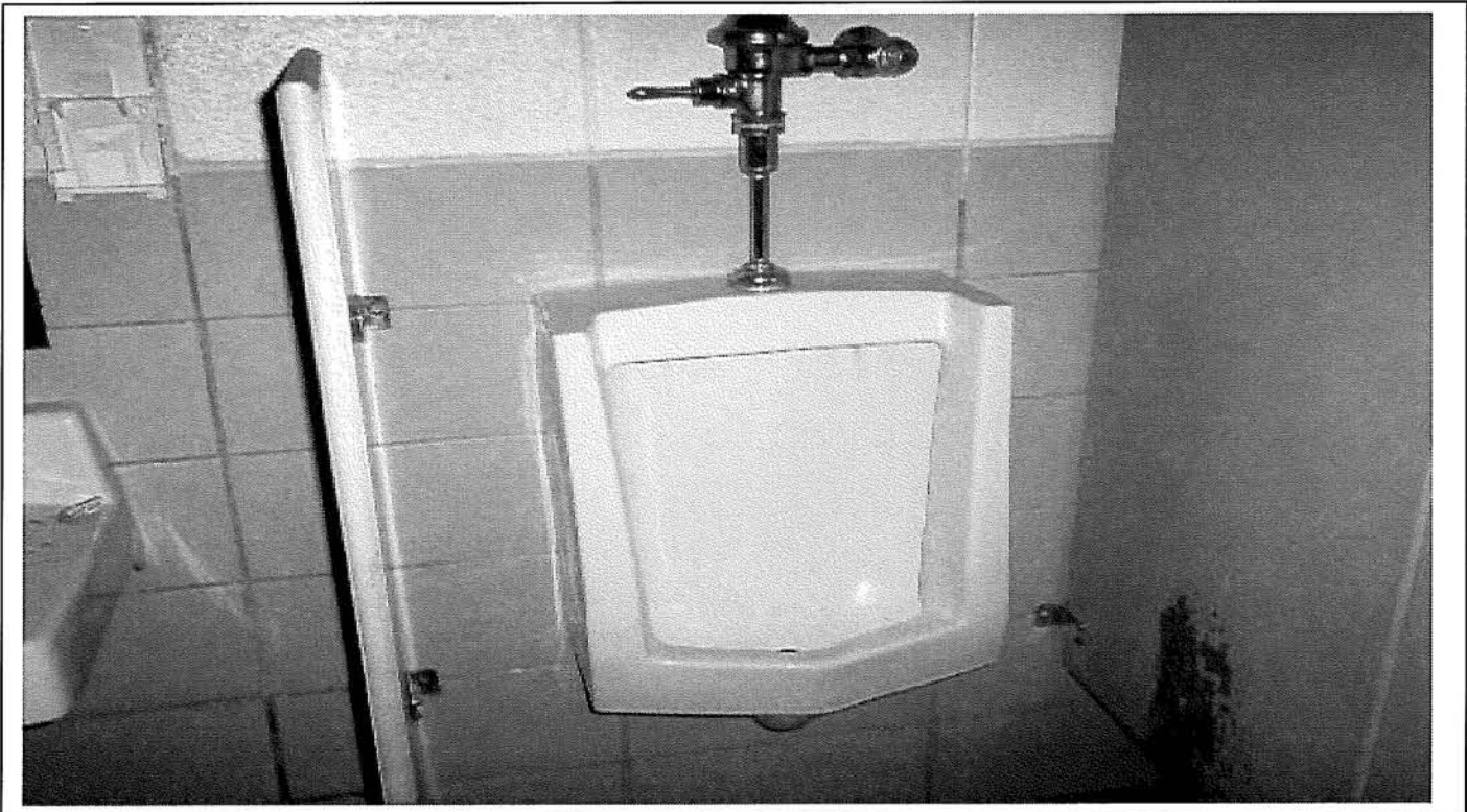
Photo 85: Typical ceramic urinal located in locker area of section 6, Therapy Building.
