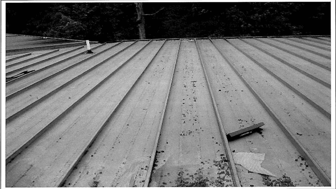
Photo 67: Typical metal raised rib roof.
