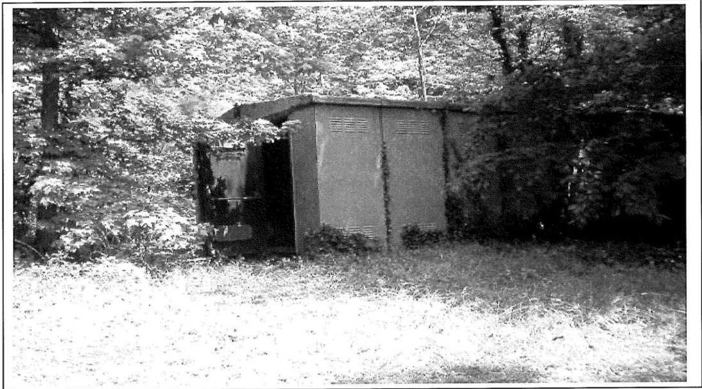
Photo 14: Miscellaneous metal storage building located behind cottage No 3.
