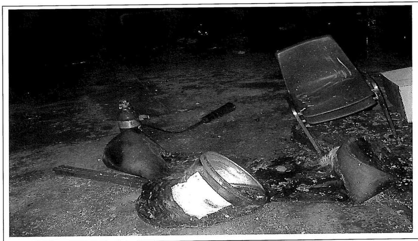
Photo 12: Debris observed in Power Plant.
