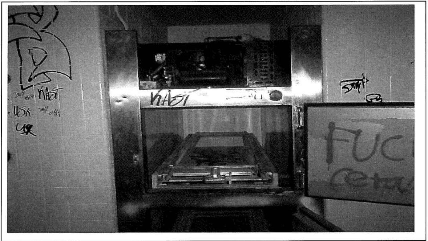
Photo 99: Typical stainless steel drawers in the morgue area, located in section 4, lower level of Therapy building.
