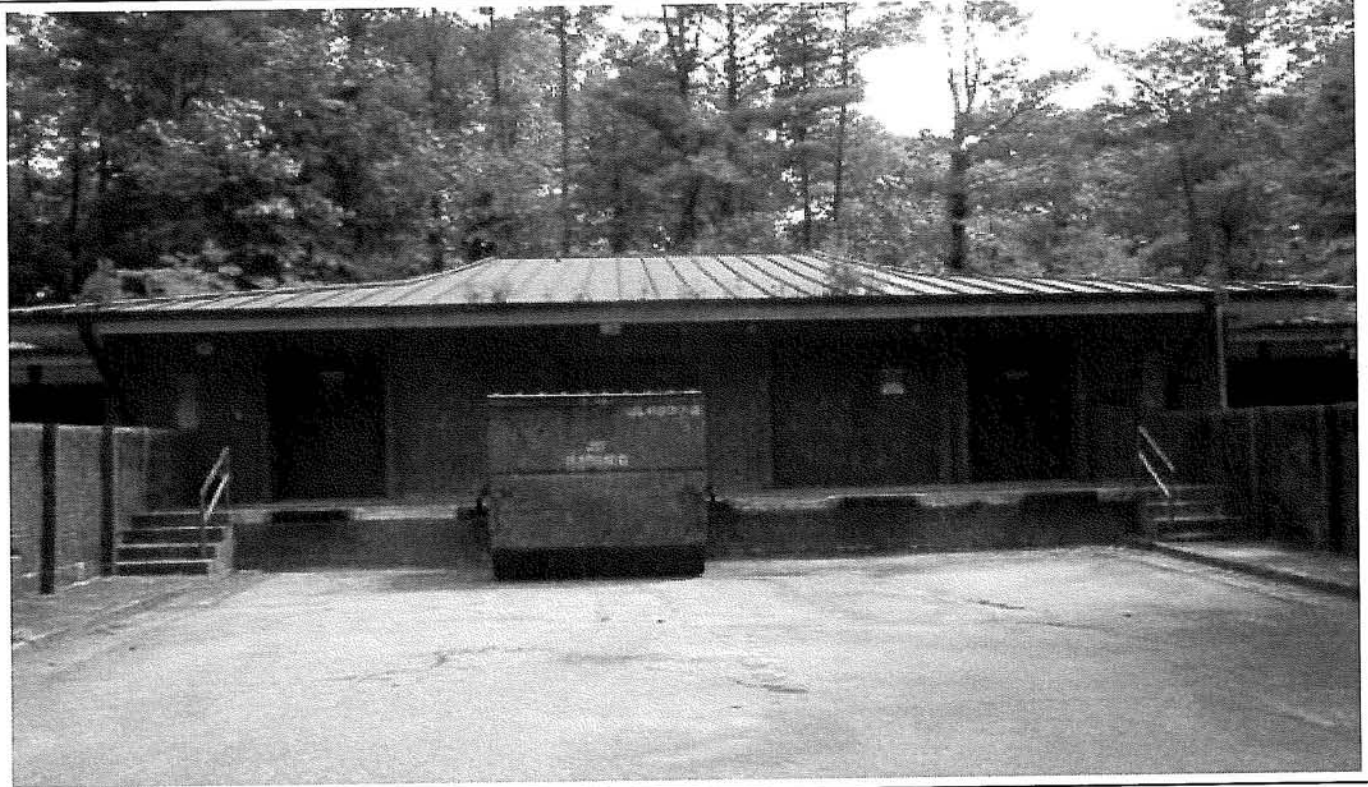
Photo 23: Typical view of cottage No. 5, loading dock area.
