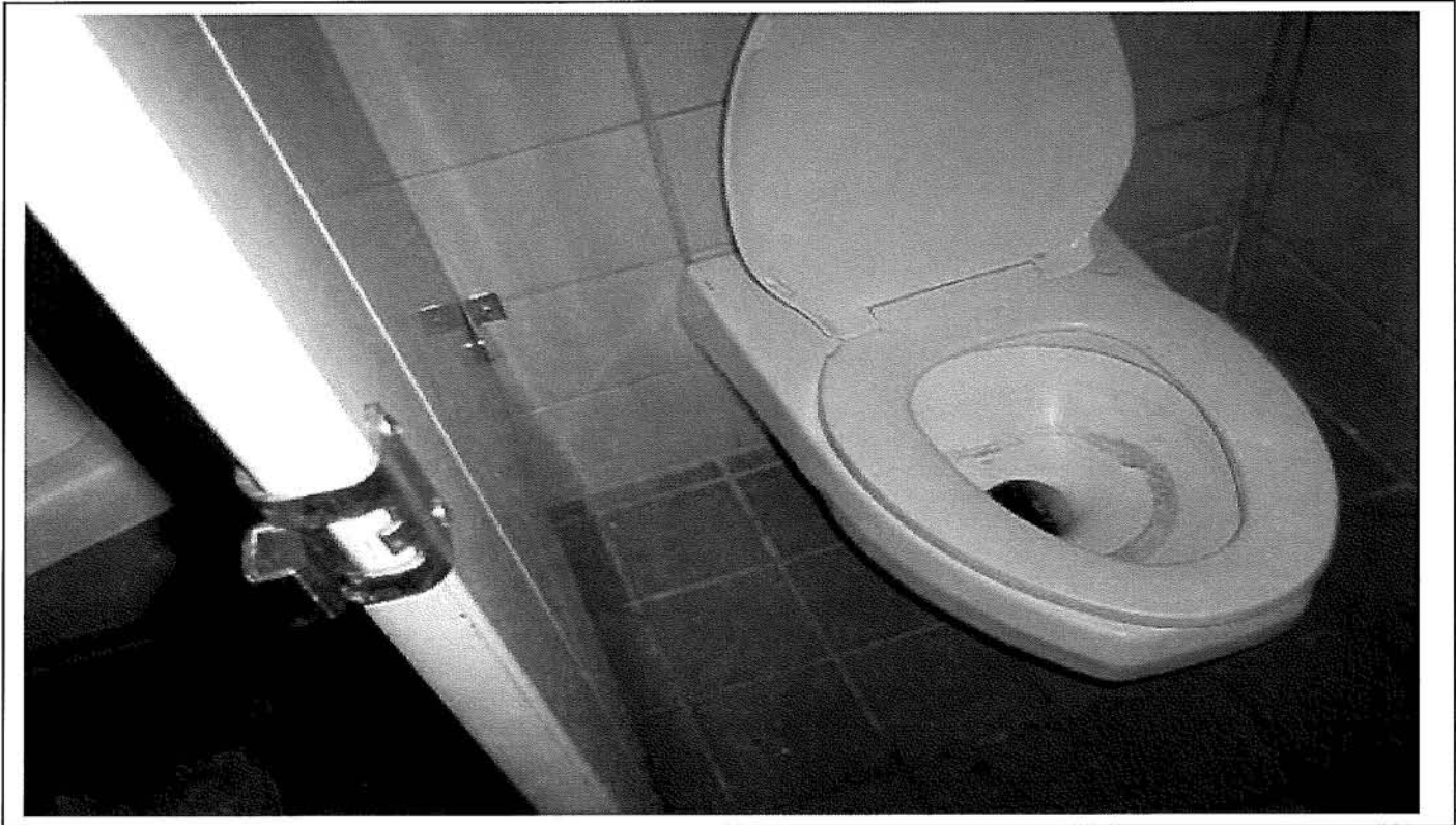
Photo 86: Typical commode located in locker area of section 6, Therapy Building.
