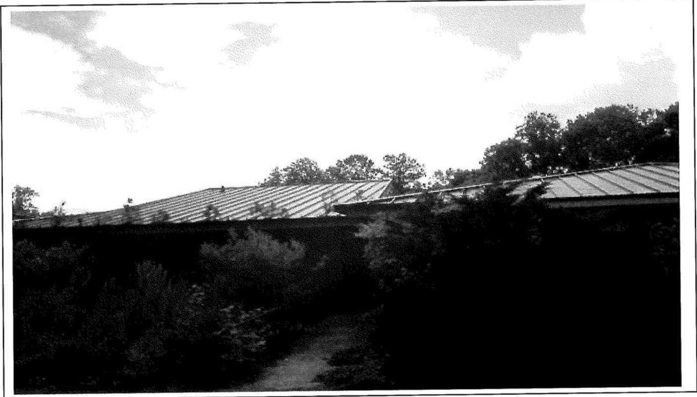
Photo 17: Typical metal standing seam roof located in cottages 3, 4 & 5.
