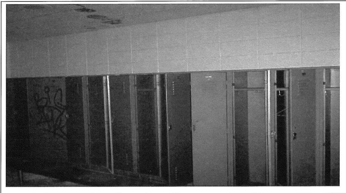
Photo 83: Typical metal lockers in locker room, located in section 6, Therapy Building.
