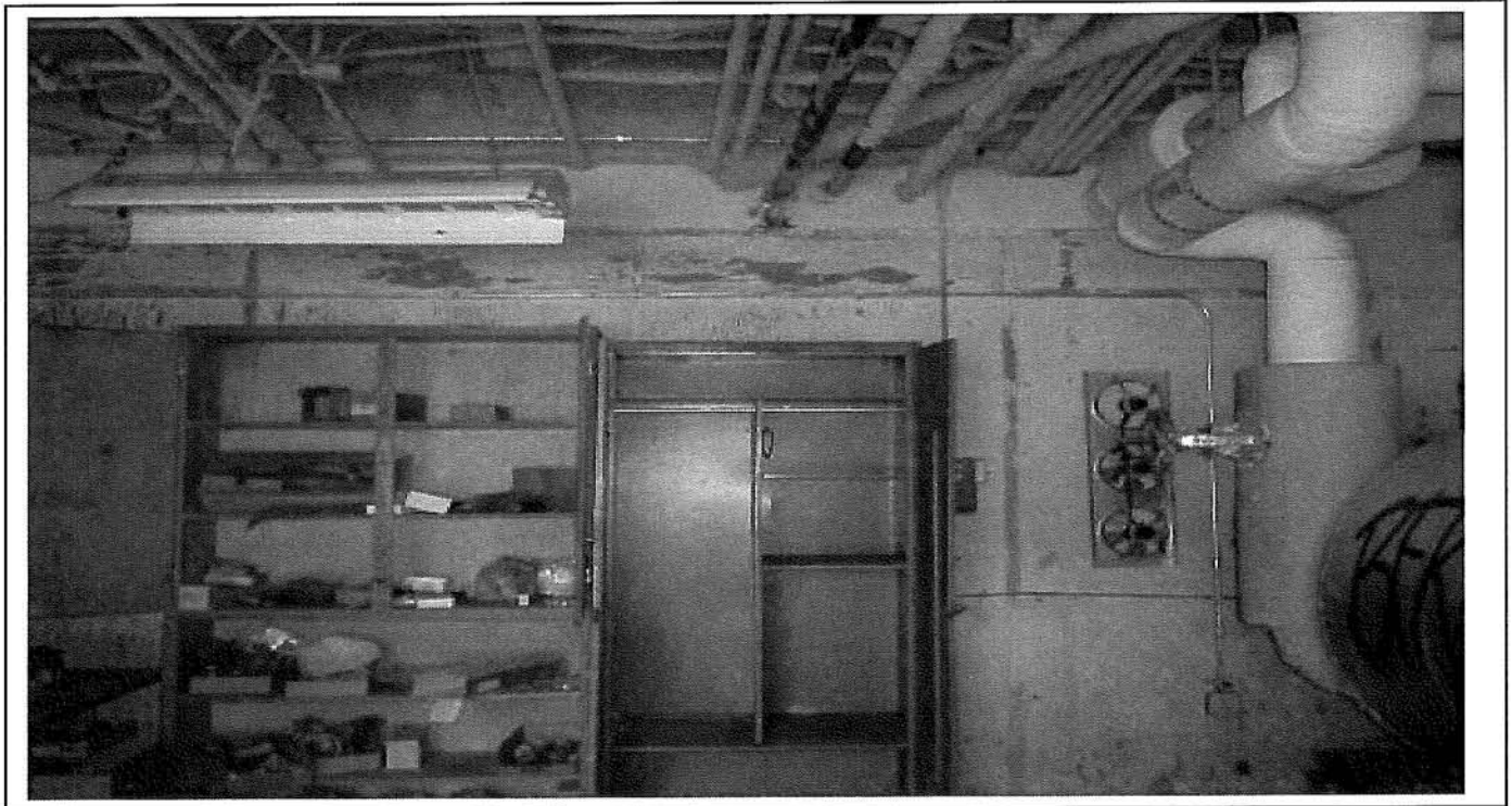
Photo 77: Metal storage cabinet located in mechanical room of section 6, Therapy Building.
