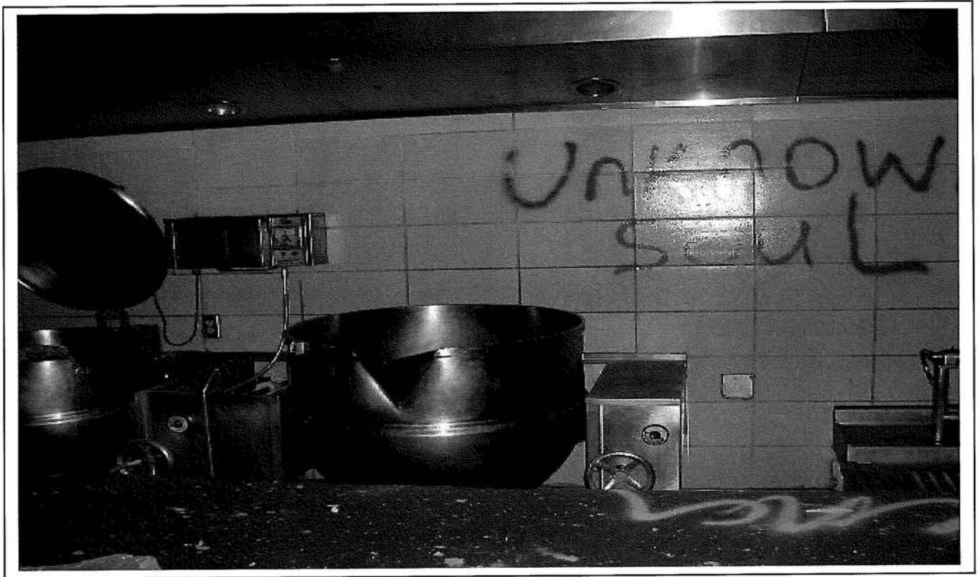
Photo 47: Typical wall-mounted deep fryers in kitchen area Therapy Building.
