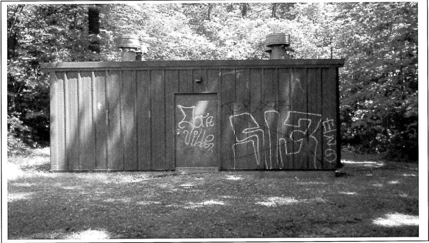
Photo 13: View of an electrical switch building adjacent cottage No 3.
