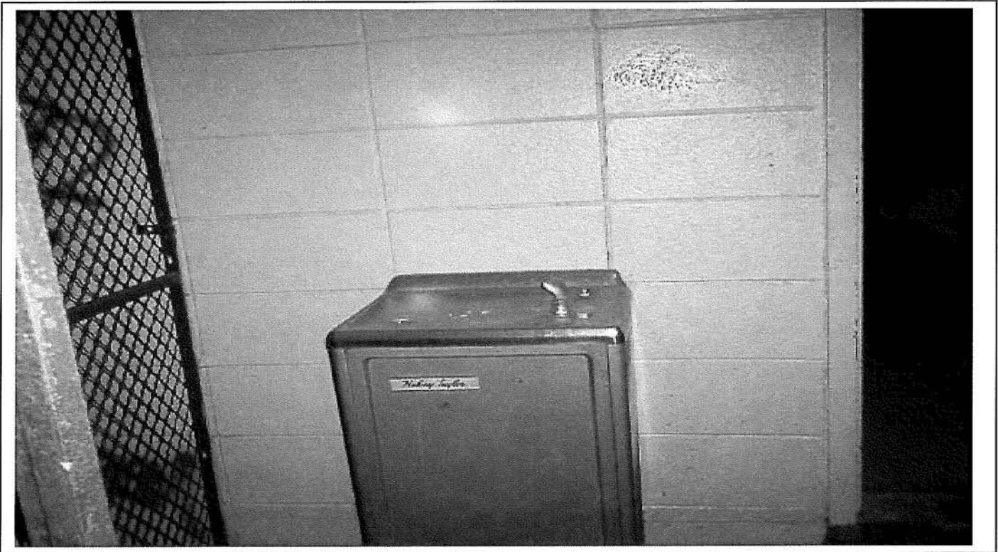
Photo 87: Typical metal wall-mounted water cooler located in storage area of section 6, Therapy Building.
