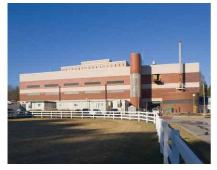
The Animal Health Research Center (AHRC) is an existing building, located on the campus at the University of Georgia in the College of Veterinary Medicine. The AHRC is a three-story concrete and masonry structure with a gross area of 72,945 SF. Construction was halted in 1998, and the building has never been commissioned for operation because of construction and operational deficiencies. The project scope involves the following elements:
