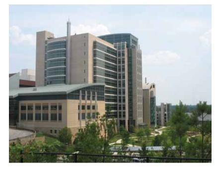
The Emerging Infectious Diseases Building is a 368,250 SF concrete structure that houses bio-safety level (BSL) 2, 3, 3E, and 4 laboratories and support spaces. The building expands CDC's BSL3 and BSL4 capacity, provides core labs for bio-terrorism, Q-fever, infectious disease and contains an animal facility. The project also included a 54,955 SF Central Energy Plant that houses chillers, cooling towers, boilers and associated pumps for the west portion of the CDC Roybal Campus.
