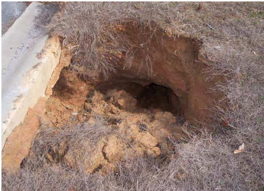
Photograph 8: View of pit located on the Subject Property.
