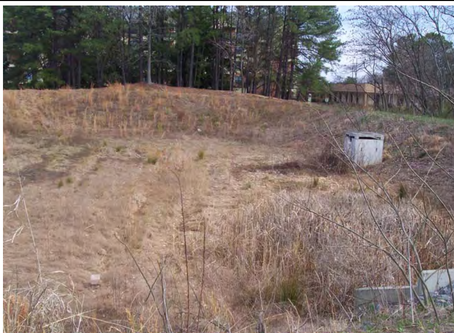
Photograph 9: View of storm water pond located on the Subject Property.
