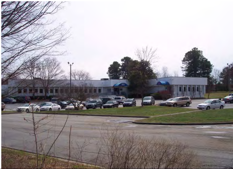
Photograph 5: View of south adjoining property.
