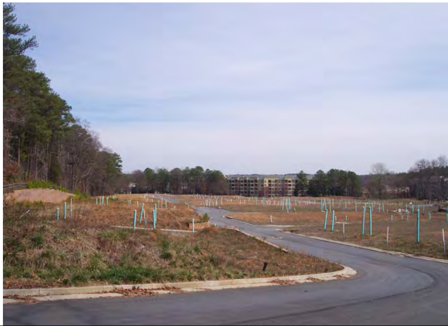
Photograph 1: View of Subject Property.
