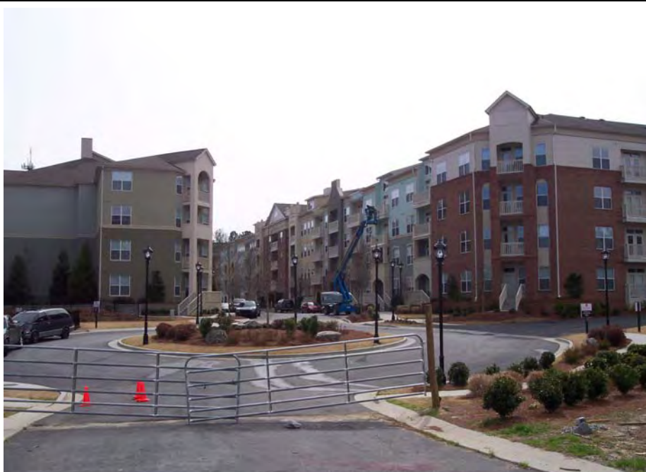
Photograph 6: View of south adjoining property.
