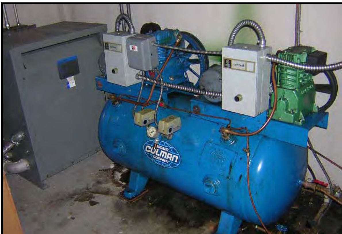
PHOTO 19 Air compressor in second floor utility room
