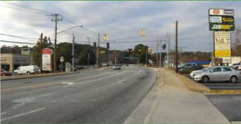
Chamblee Dunwoody Road- Today
