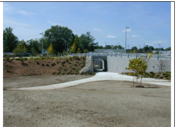
WMU Pedestrian Underpass (The CSM Group)
