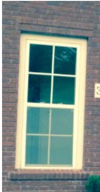
WINDOW W/ BRICK SILL & HEADER
