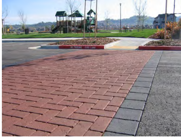
Stamped asphalt crosswalk
