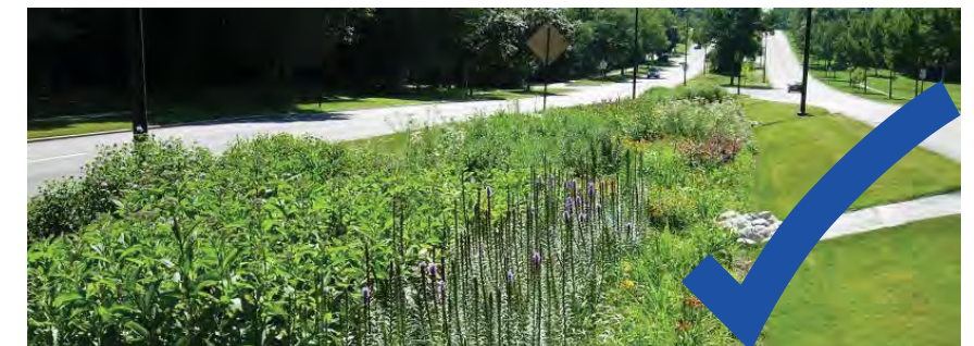
2. Bioretention Area Between Roadways
