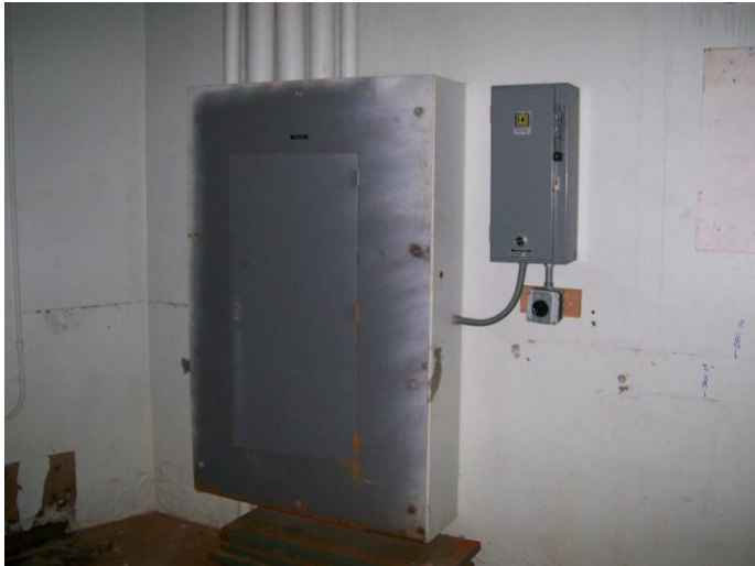
Water Damage at Main Distribution Panel “PP-L”
