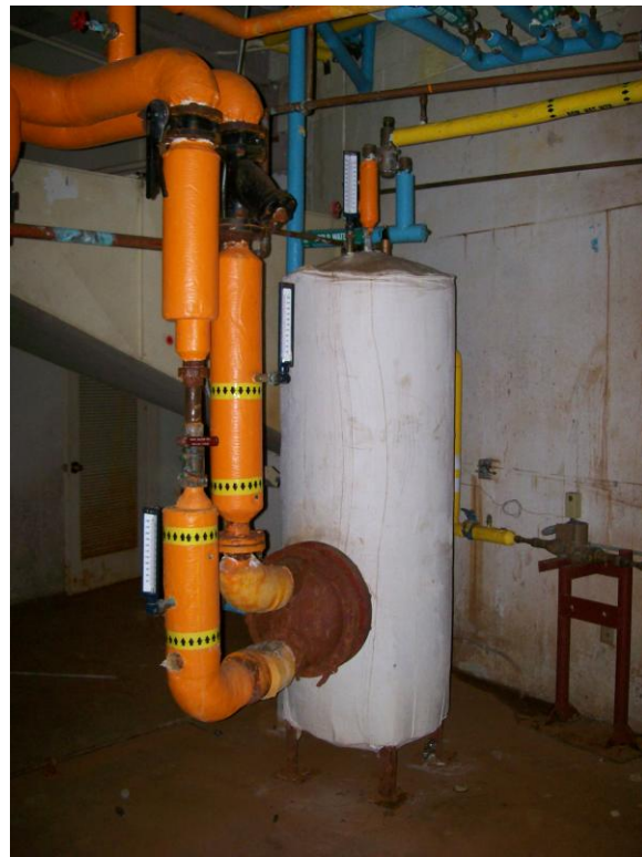
Domestic Water Heat Exchanger
