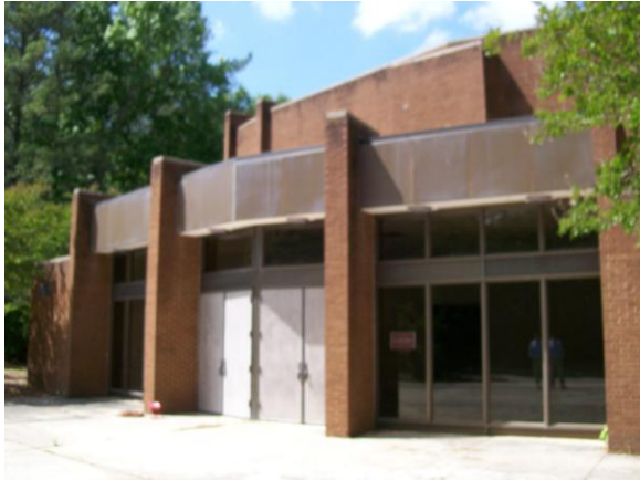
Main Entry of Theater
