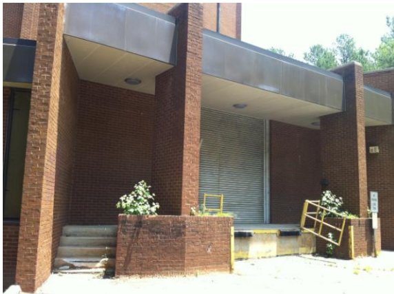
Loading Dock at Rear of Facility
