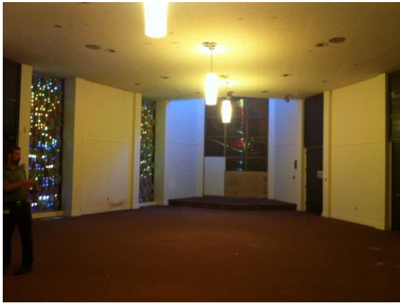
Vandalism at Chapel Windows
