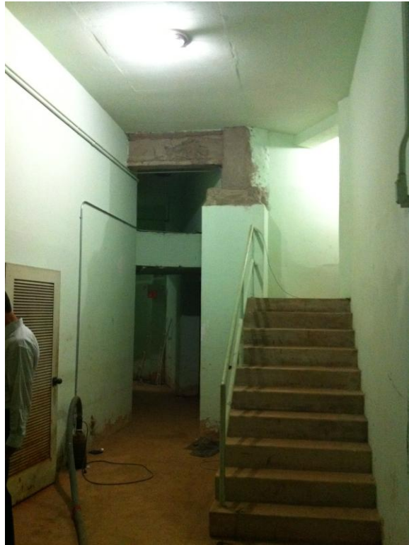
Basement Corridor and Stair
