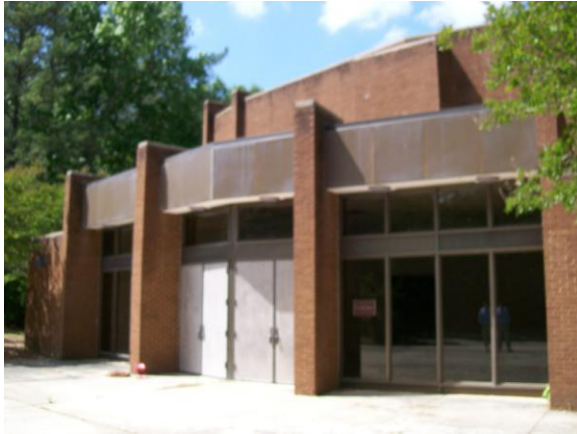
Main Entry of Theater
