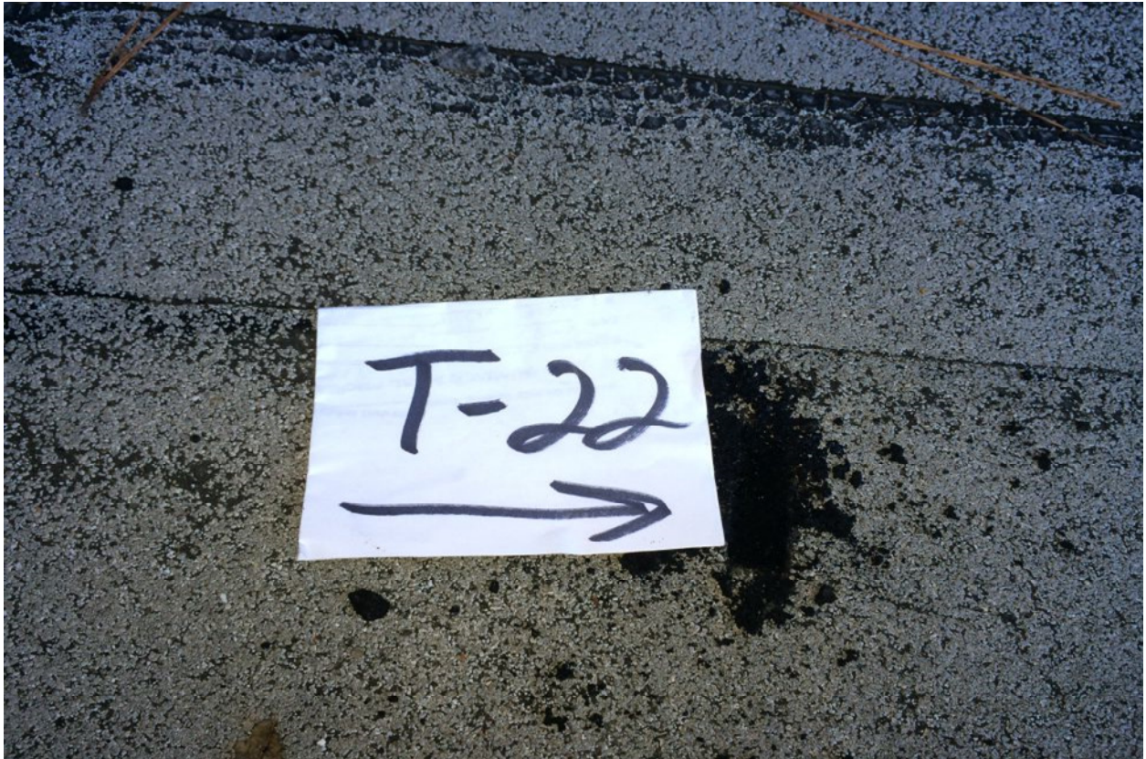
Plate 71: Laboratory analyses did not detect asbestos minerals within asphalt roof sample TS-22 collected from the Theatre Building roof.
