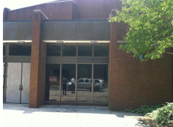
Original Glazing in Aluminum Storefront
