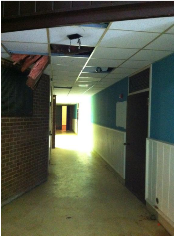
Typical Condition at Corridors
