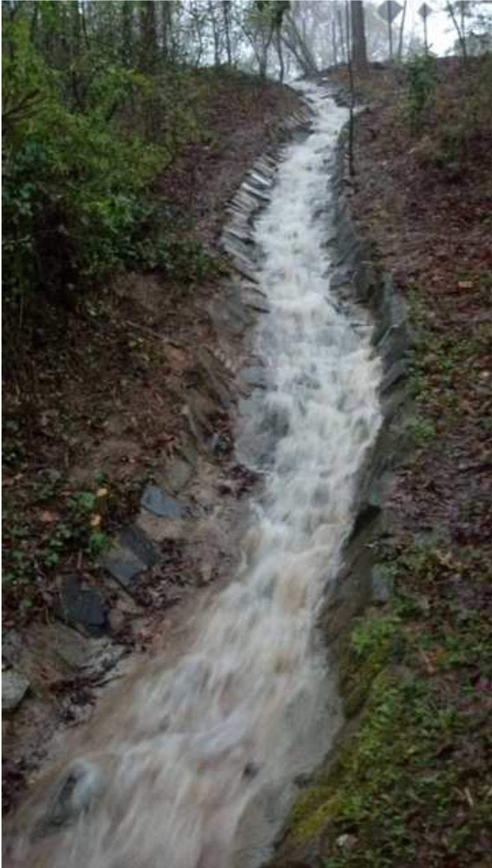
Flume leading from Bentbrook Drive to be abandoned
