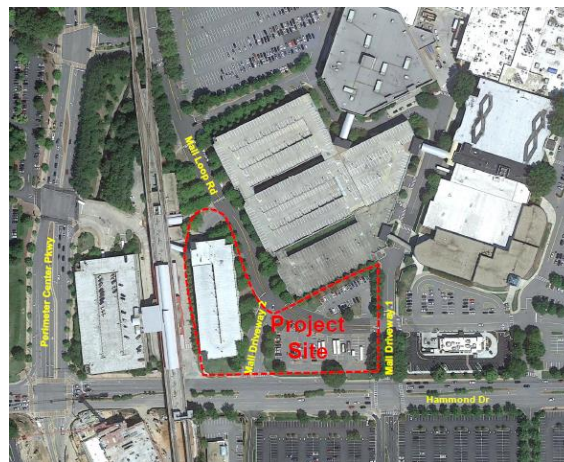
Figure 1: Project Site Aerial
