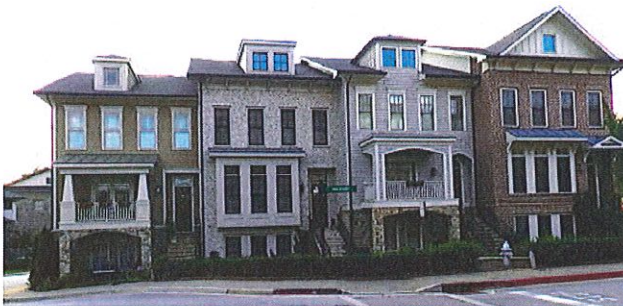
Figure 27-98-34 Examples of Ground Story along Slope.
