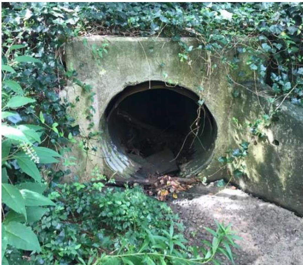
Excess debris, and misalignment at headwall
