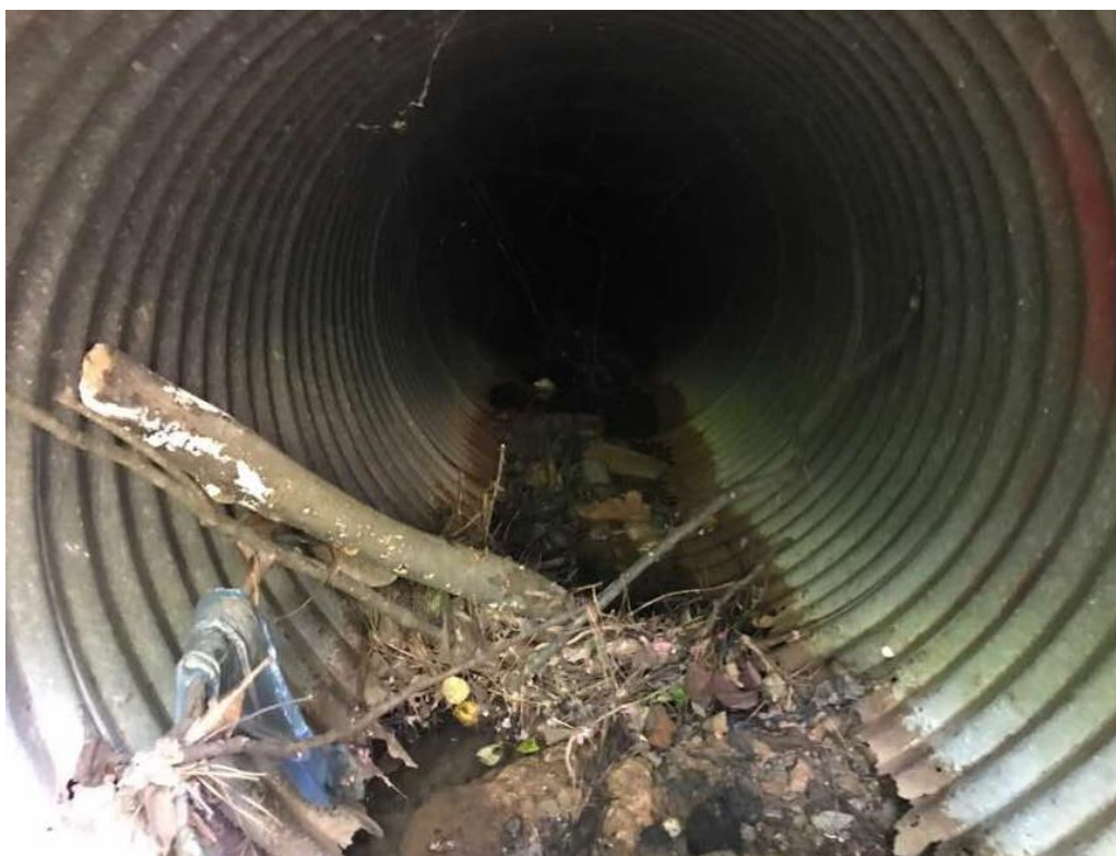
Invert Failure, excess debris in 42" CMP
