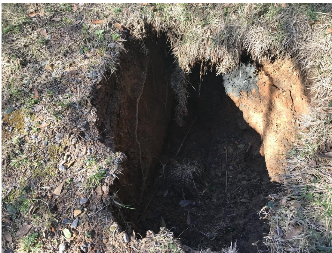
Sinkhole Formation Due to Pipe Failure
