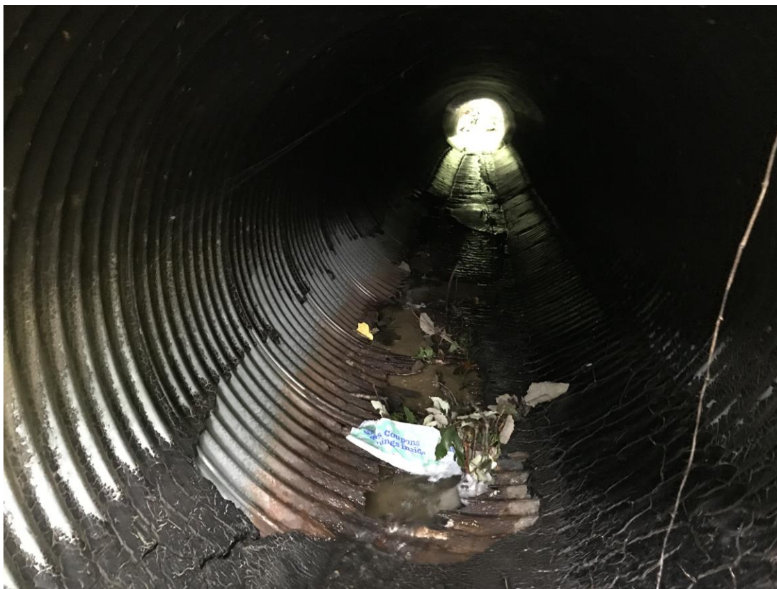
Invert failure of Corrugated Metal Pipe
