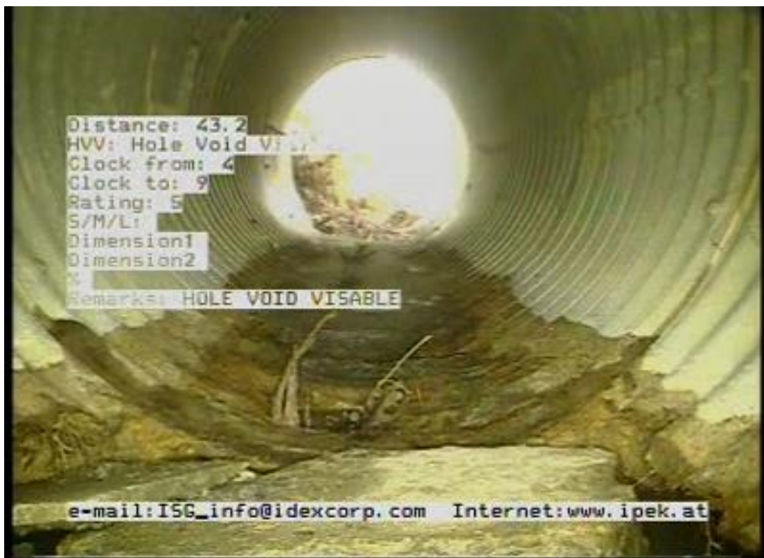
Pipe Invert Failure and Visible Hole
