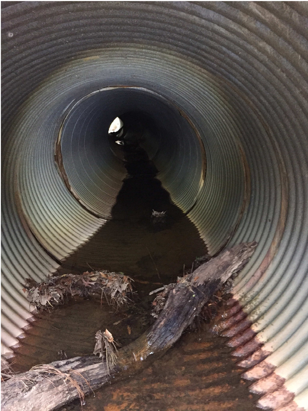
Invert Failure and Poor Alingment Throughout Pipe
