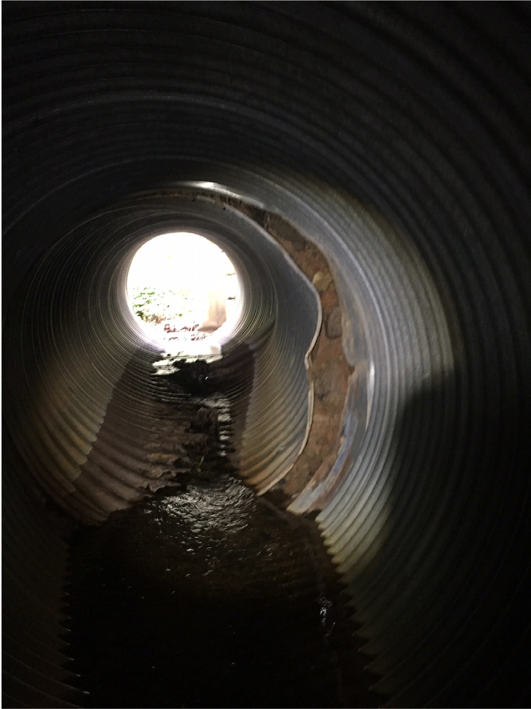
Pipe Joint and Invert Failure Causing Primary Sink Hole
