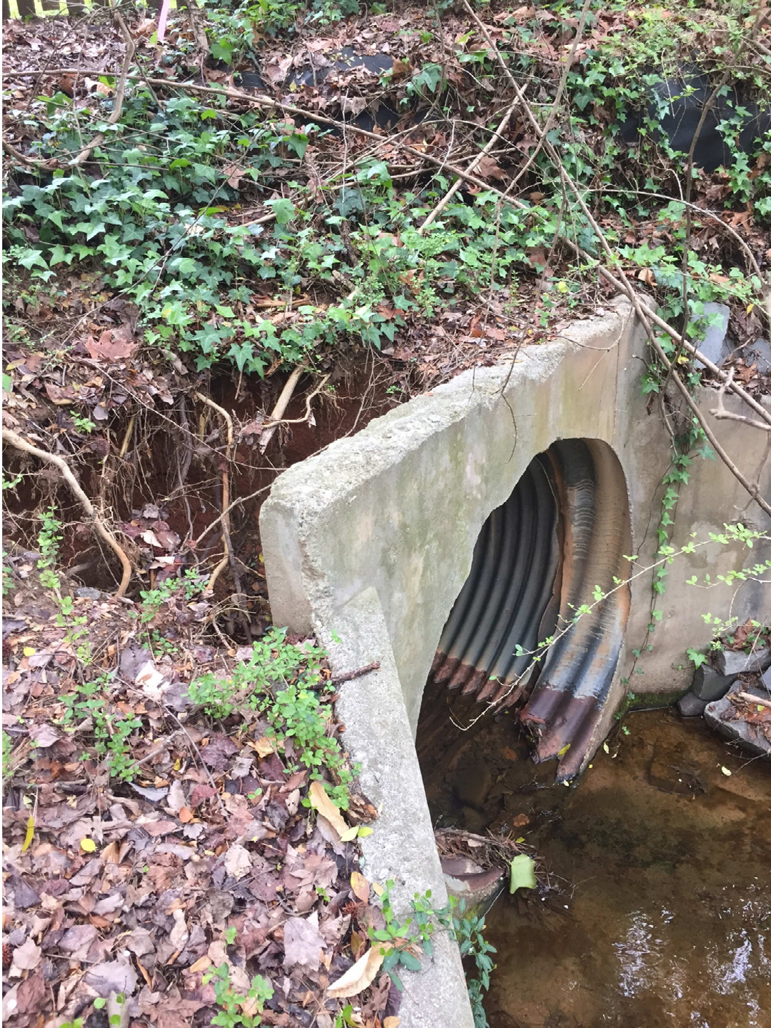
Pipe and Headwall Failure at Downstream End of Culvert
