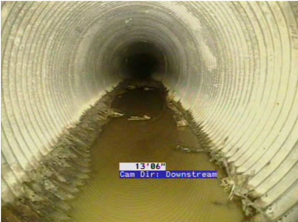
Rusted and Missing Pipe Invert Causing Sink Holes
