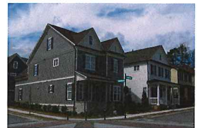
▲ New Housing in Georgetown
