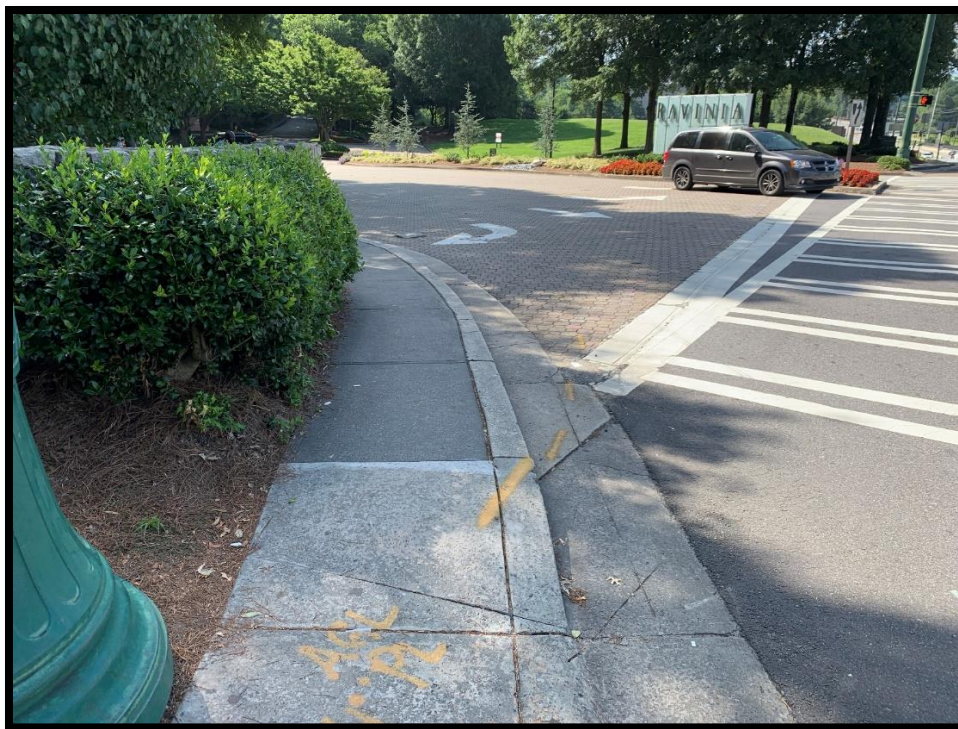
Photograph 2 – Narrow Sidewalk and Lack of Lane Striping in Northeast Corner of Ashford Dunwoody at Ravinia
