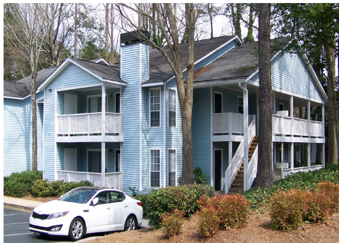
▲ Apartments off of North Peachtree Road
