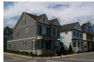
▲ New Housing in Georgetown
