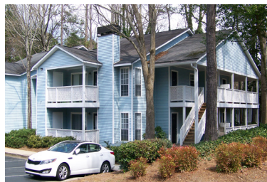
▲ Apartments off of North Peachtree Road
