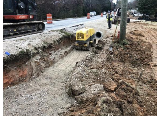
Tilly Mill Road Sidewalk- Stormwater Pipe Installation
