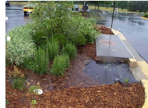
Middle Right: Figure 4.2-4 Bioretention Area after Storm
