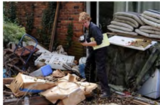
Stone Mountain, GA, October 22, 2009 -- Lorie Cornwell, a volunteer with DeKalb Emergency Management Agency, inspects a flood damaged residence in DeKalb County. The site visit is part of a county-sponsored training class for area officials on how to evaluate damaged houses, using a new FEMA software program that makes it easier for communities to assess residences
