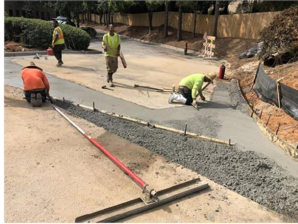
Driveway Replacement North Shallowford
