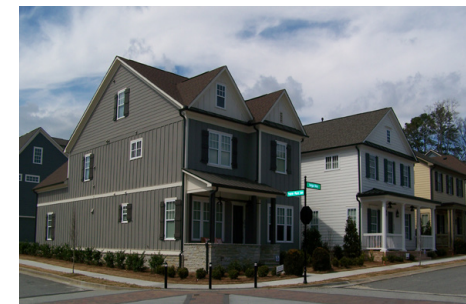
▲ New Housing in Georgetown
