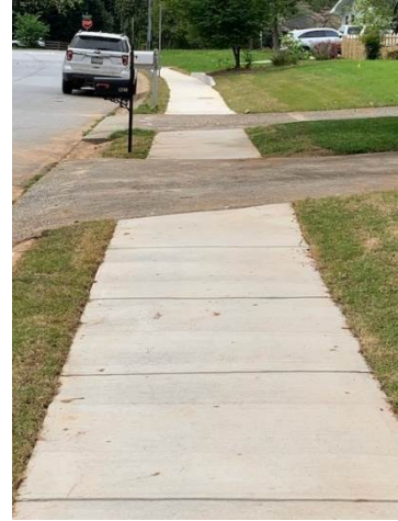
Completed Sidewalk on Olde Village Run
