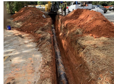
Georgetown Water Main Installation
