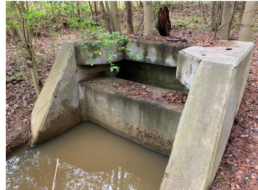
EXISTING BAFFLED INLET
