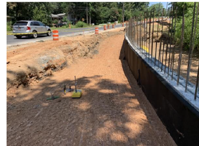
Retaining Wall near Georgetown Park
