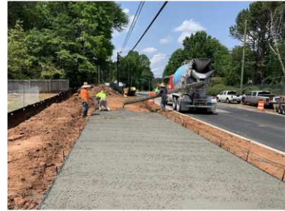
Winters Chapel New Curb
