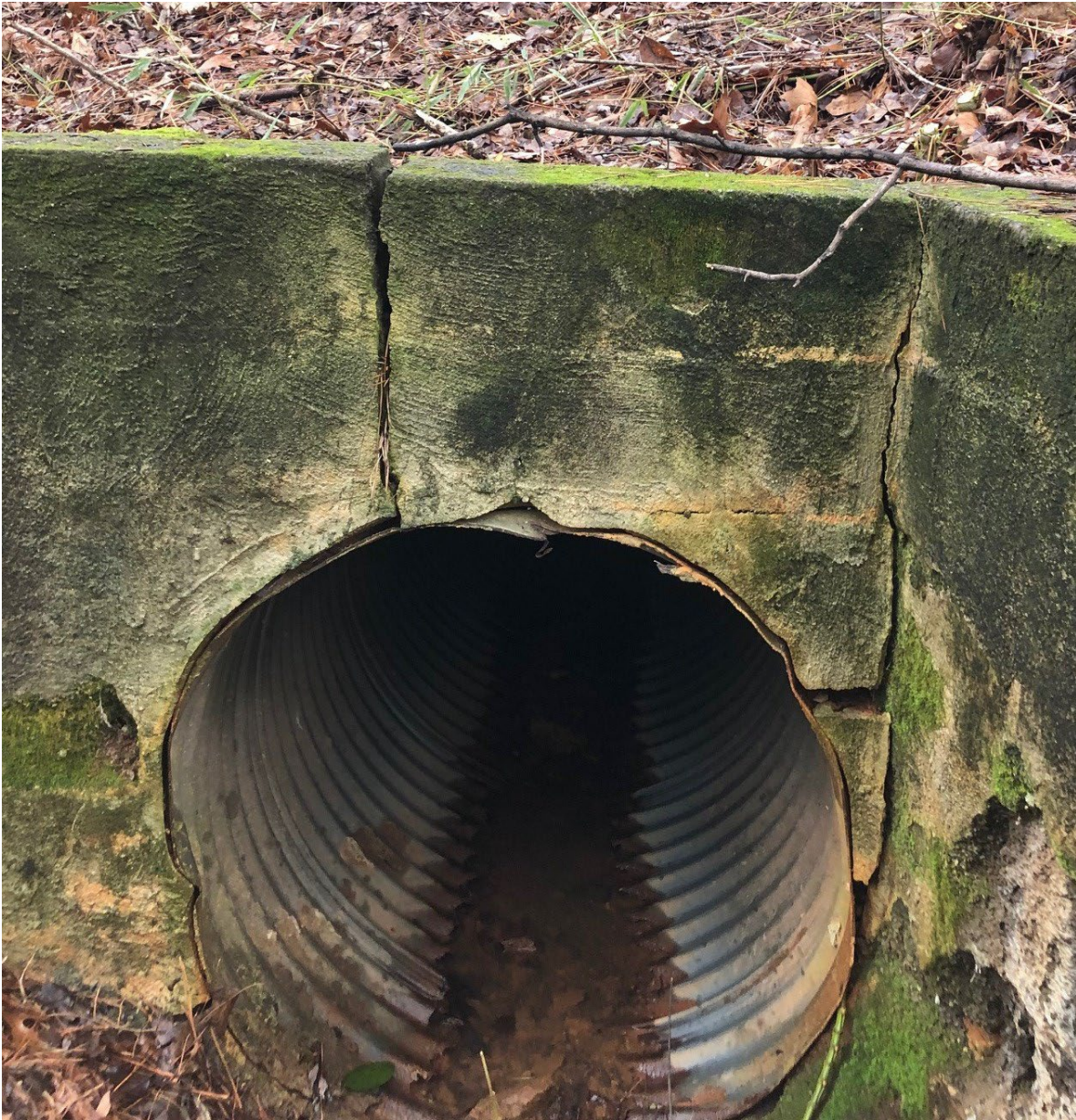
Damaged Outlet Headwall
