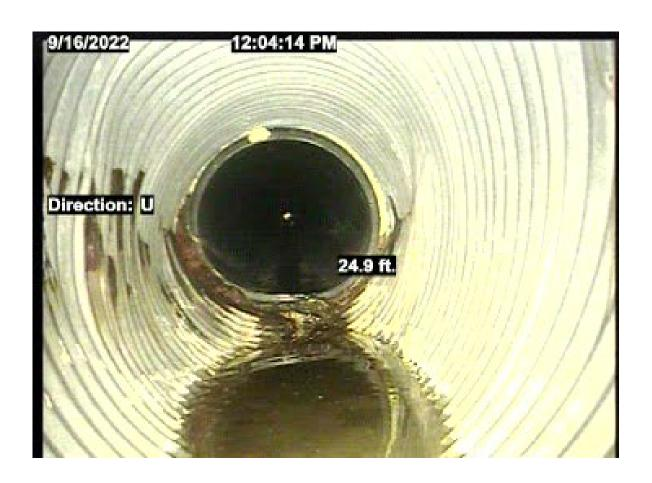
Partial slip-line under driveway, joint separation, and deformities
