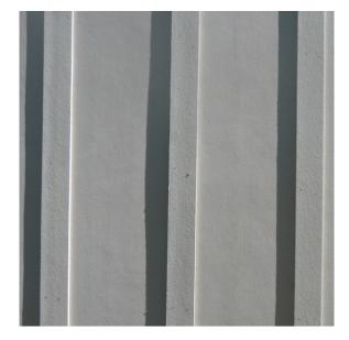
FIBER CEMENT PANELS -BOARD AND BATTEN
