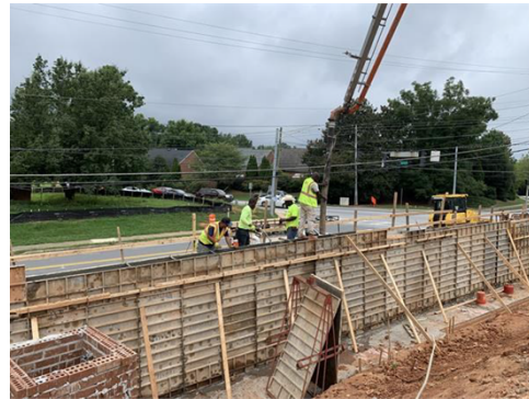
Wall Construction on Womack Road
