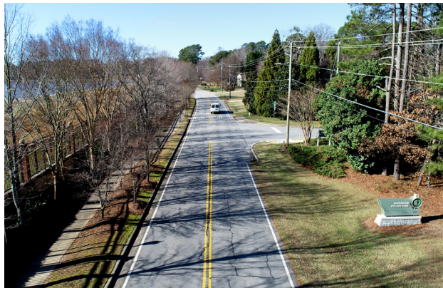
Existing conditions of Peeler Road, looking west.
