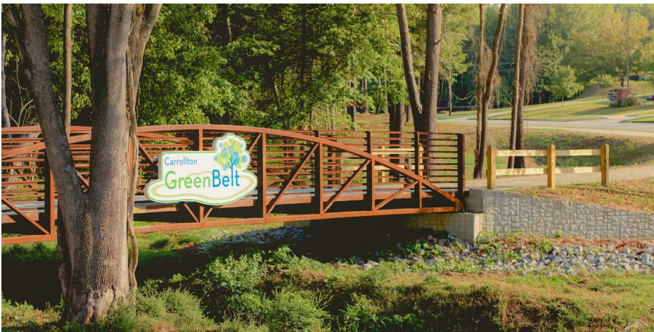
Prefabricated steel bridge allows the trail to cross above existing roads and waterways.
