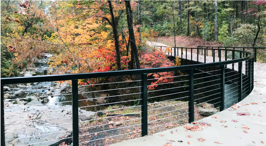
Bridges with painted finishes are timeless and suitable for urban environments
