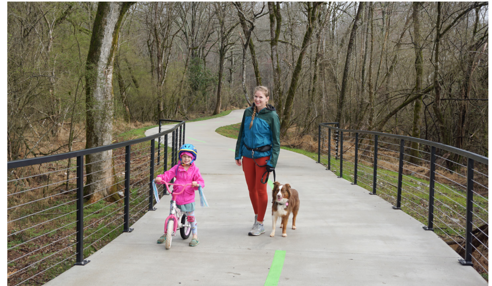
Concrete boardwalk structures built with top-down construction methods provide durable, minimally invasive, and ecologically sensitive trail connections through wetlands and established forests.
