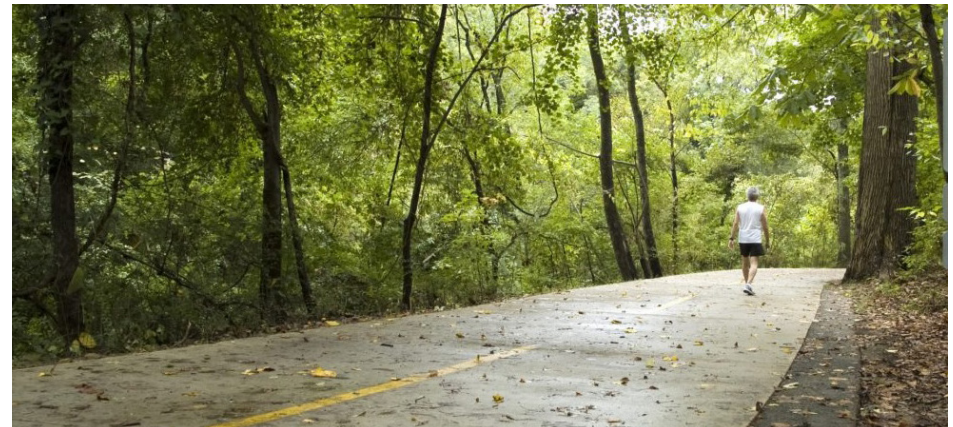
Tree root bridging allows the trail to come close to specimen trees without causing harm. A trail edge of porous concrete aids infiltration.
