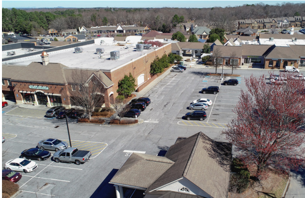
Existing Dunwoody Village parking lot, looking northeast.
