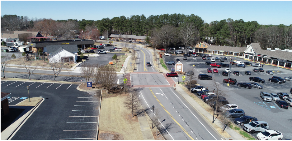
Looking north of the existing conditions on Dunwoody Village Parkway
