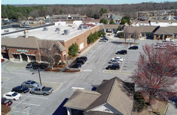
Existing Dunwoody Village parking lot, looking northeast.
