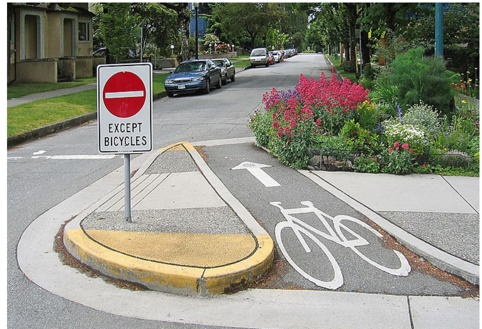
Calm Streets example showing limited vehicle entry while utilizing signage and pavement markings for bicycle riders.
