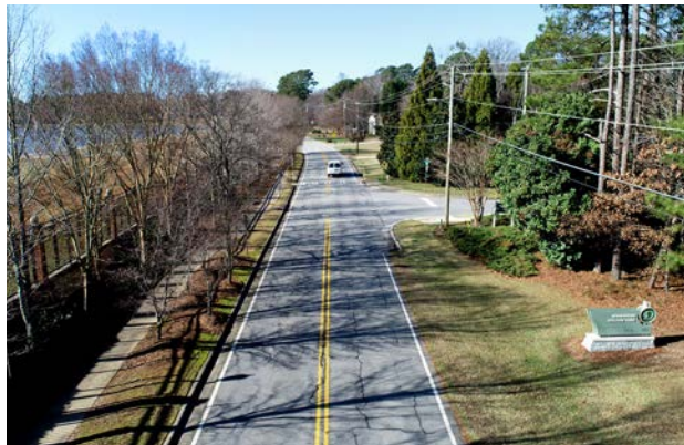
Existing conditions of Peeler Road, looking west.
