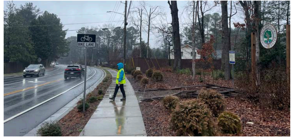
Existing sidewalk and bike lane at the Roberts Drive entrance to the Nature Center
