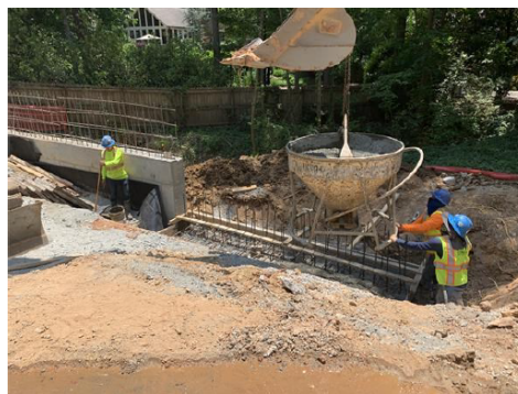
Dunwoody Road Wall Construction
