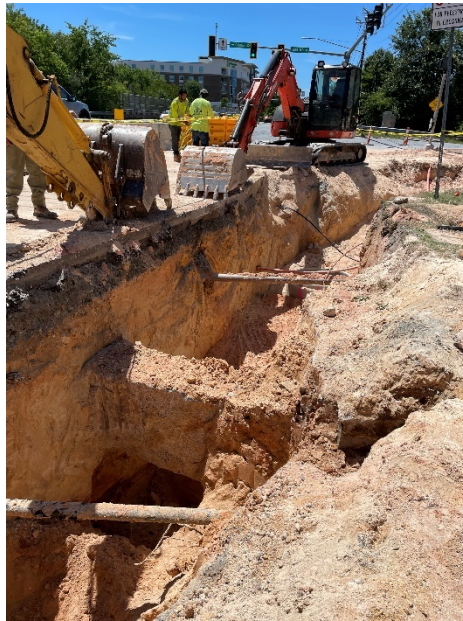
Georgetown Gateway Stormwater Pipe Installation
