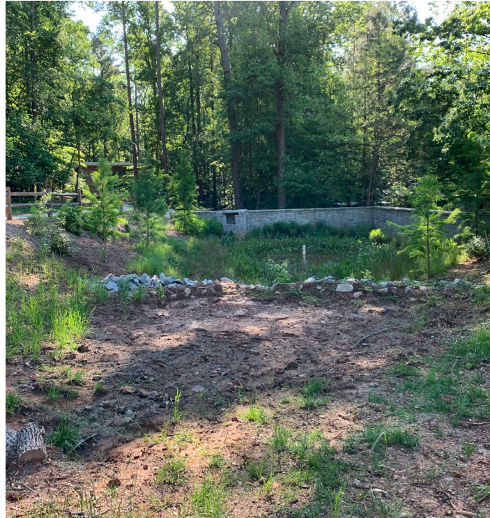
View looking down drainage swale into existing rain garden.
