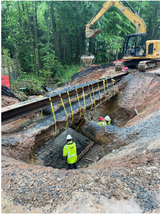
Dunwoody Road Wall Construction
