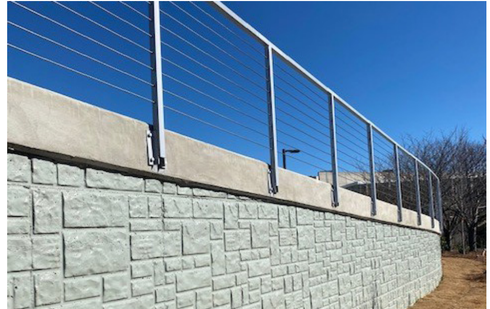
Post and cable railing provides a safe trail edge while acting as a visually lighter option.
