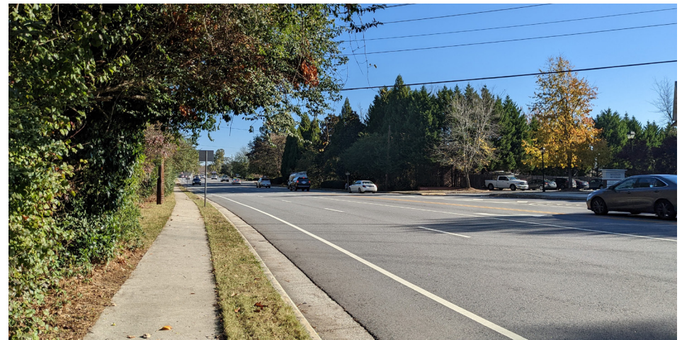
Existing sidewalk and bike lane on Mount Vernon Road east of the intersection with Ashford Dunwoody Road
