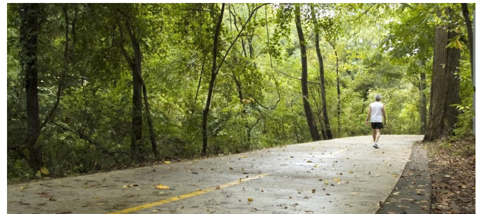
Tree root bridging allows the trail to come close to specimen trees without causing harm. A trail edge of porous concrete aids infiltration.
