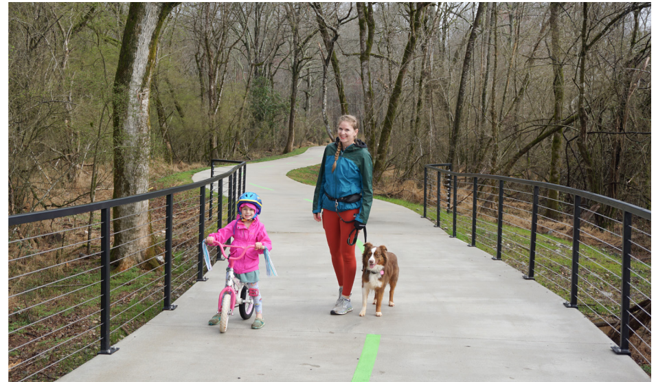
Concrete boardwalk structures built with top-down construction methods provide durable, minimally invasive, and ecologically sensitive trail connections through wetlands and established forests.
