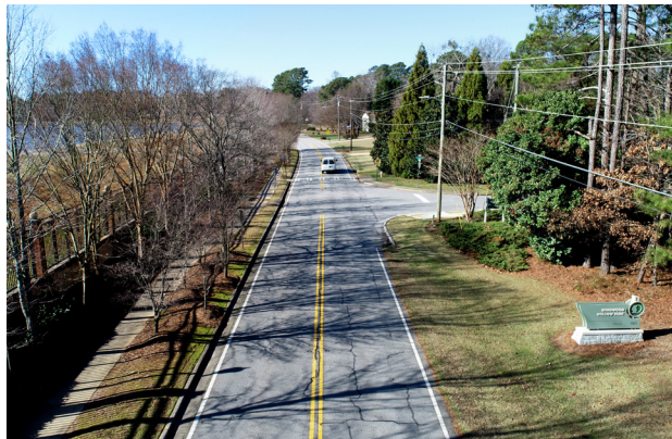
Existing conditions of Peeler Road, looking west.
