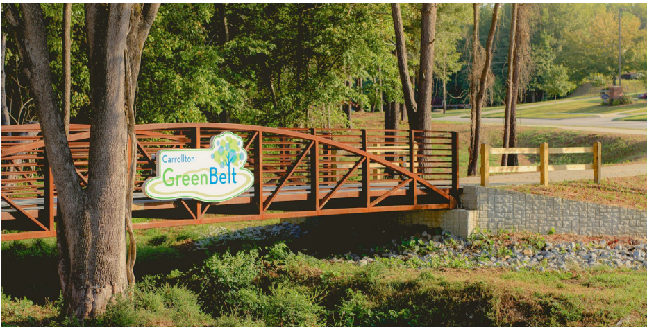
Prefabricated steel bridge allows the trail to cross above existing roads and waterways.
