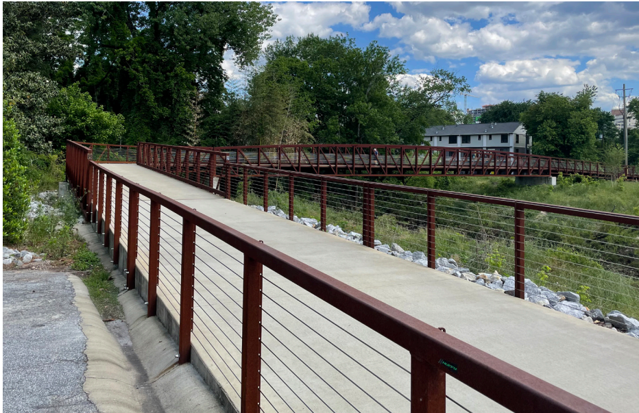
An example of the cable handrail with corten steel posts and top rail.
