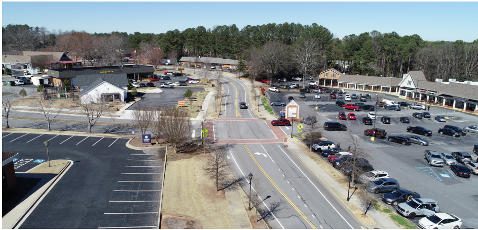
Looking north of the existing conditions on Dunwoody Village Parkway
