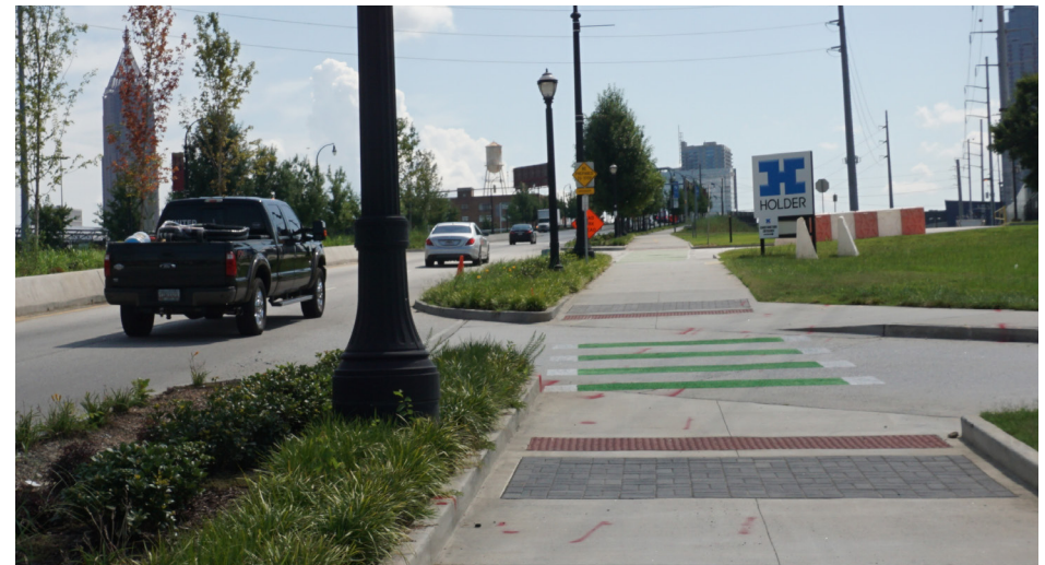
Green-striped crosswalk on Ivan Allen PATH in Atlanta, Georgia
