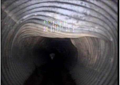
Corrosion With Visible Holes Minor Deformities To Pipe Crown
