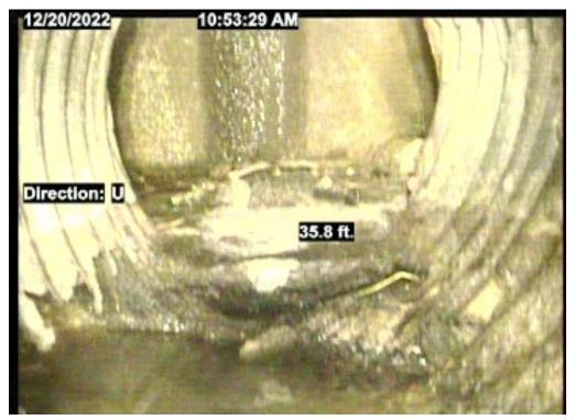
Corrosion with visible holes
