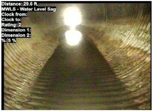
Severe Corrosion with visible holes Water Sagging
