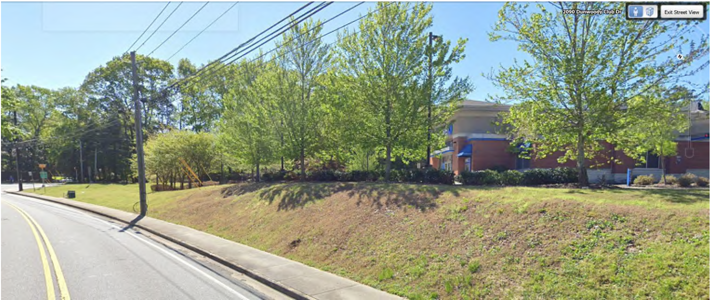
South on Jett Ferry Rd.
