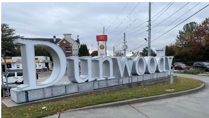
Gateway Sign at Chamblee Dunwoody Road and Cotillion Drive
