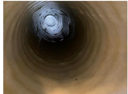
Pipelining on Coldstream Drive
